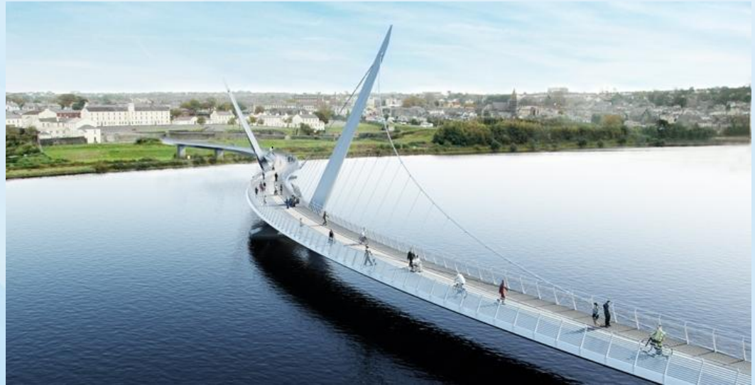
Peace bridge – Londonderry , a new and ‘iconic’ foot and cycle bridge designed to help promote greater cross-community interaction and engagement.
