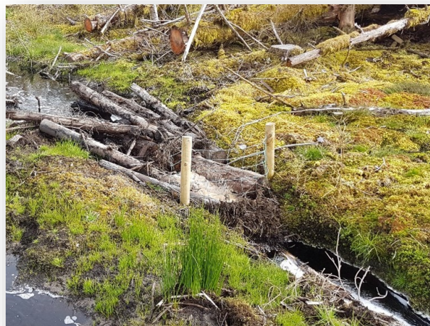
Log dam on a stream draining a Forest Service NI compartment.
