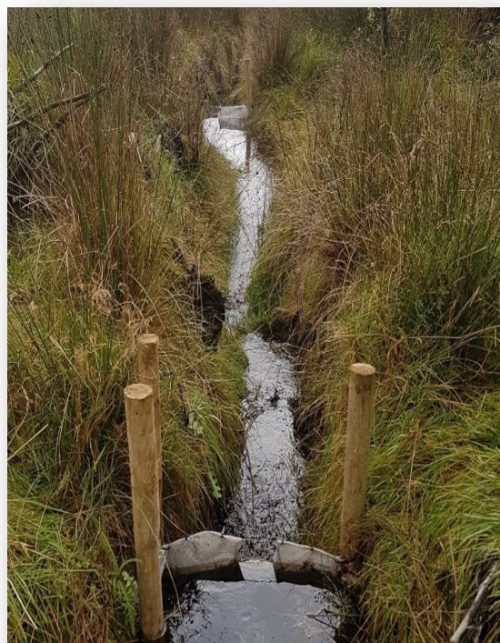
A geotextile dam installed along a watercourse draining a Coillte site.
