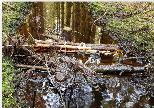
Brush dam in a small drain, draining a Forest Service NI compartment.
