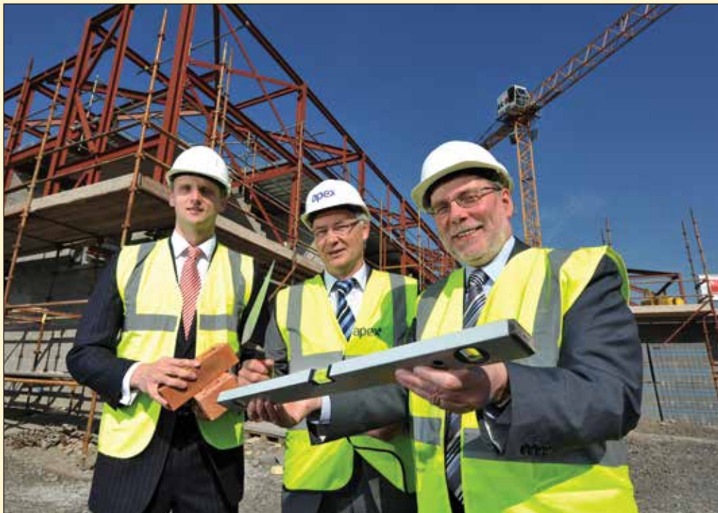
Photo Caption: (l-r) John McCandless, SEUPB, Gerry Kelly, Apex Housing and Social Development Minister Nelson McCausland, MLA take a tour of the Glen Community project construction site.
