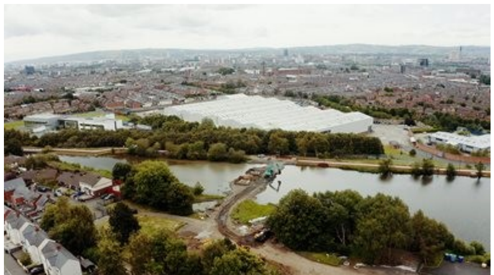
An aerial photo of the work completed to date (January 2021) at Springfield Dam.
