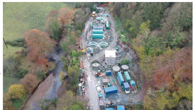
Pictured: Donemana WasteWater Treatment Works
