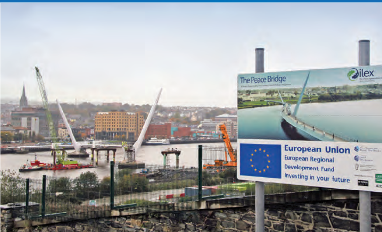
The Peace Bridge at an advance stage of its construction.
